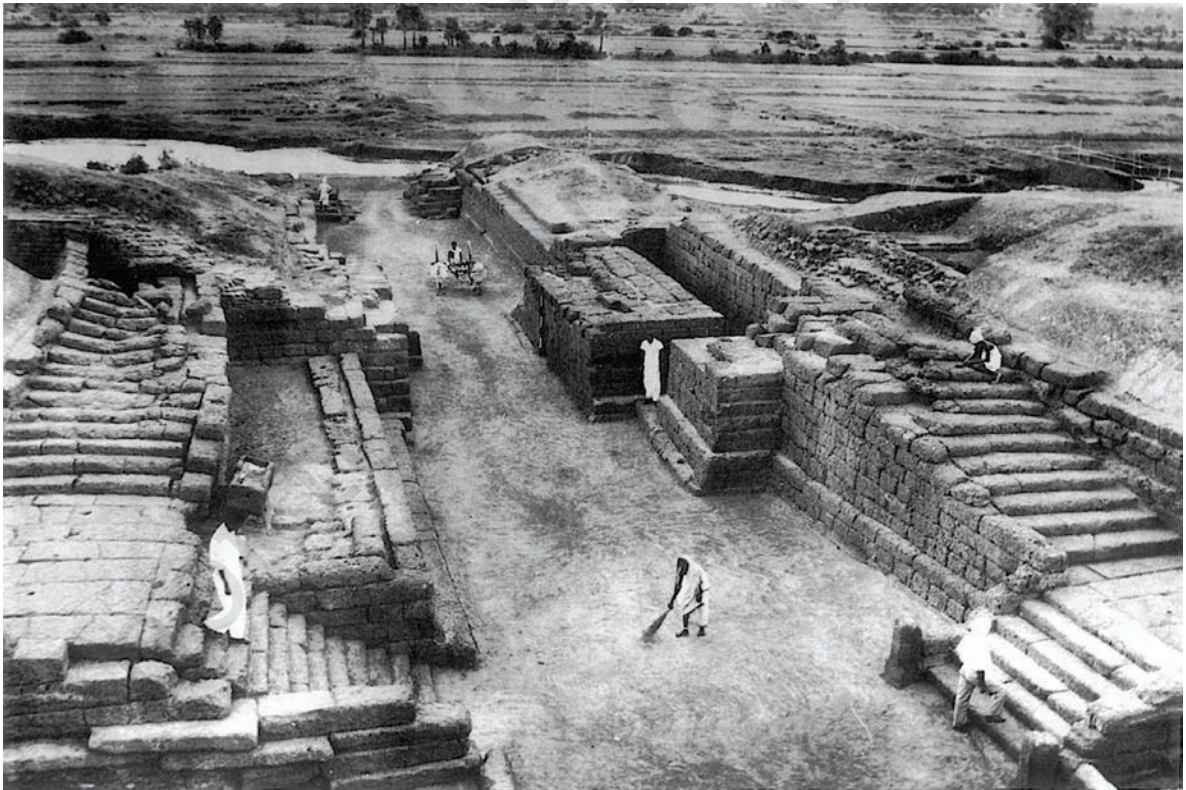
Fig. 4.7. Śiśhupalgarh (today a suburb of Bhubaneswar, first excavated in 1948): one of the gateways into the city, through the fortifications; the moat, full of water, is visible outside the gateway. Notice the narrowing in the gateway, for control of movement of people and goods.
